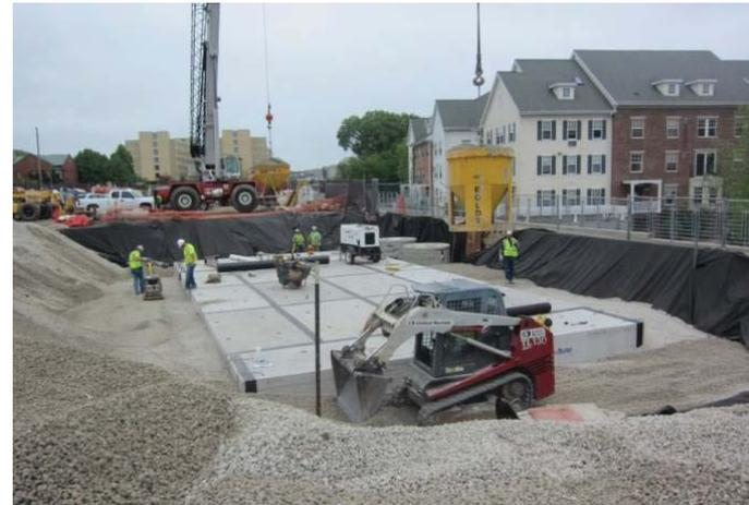
Near East Fields will utilize a similar approach by creating an underground storage facility using premanufactured vaults, pipes, or other open storage devices to detain stormwater onsite.
